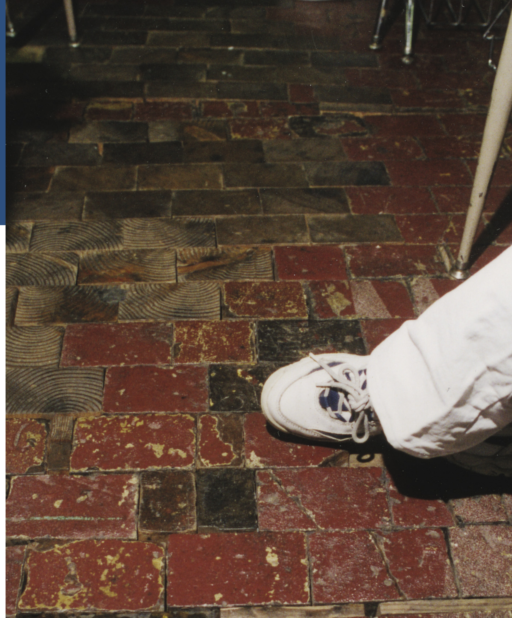
A wood-block floor of a classroom at Mark Keppel High School in Alhambra is falling apart in this 1999 photograph.
