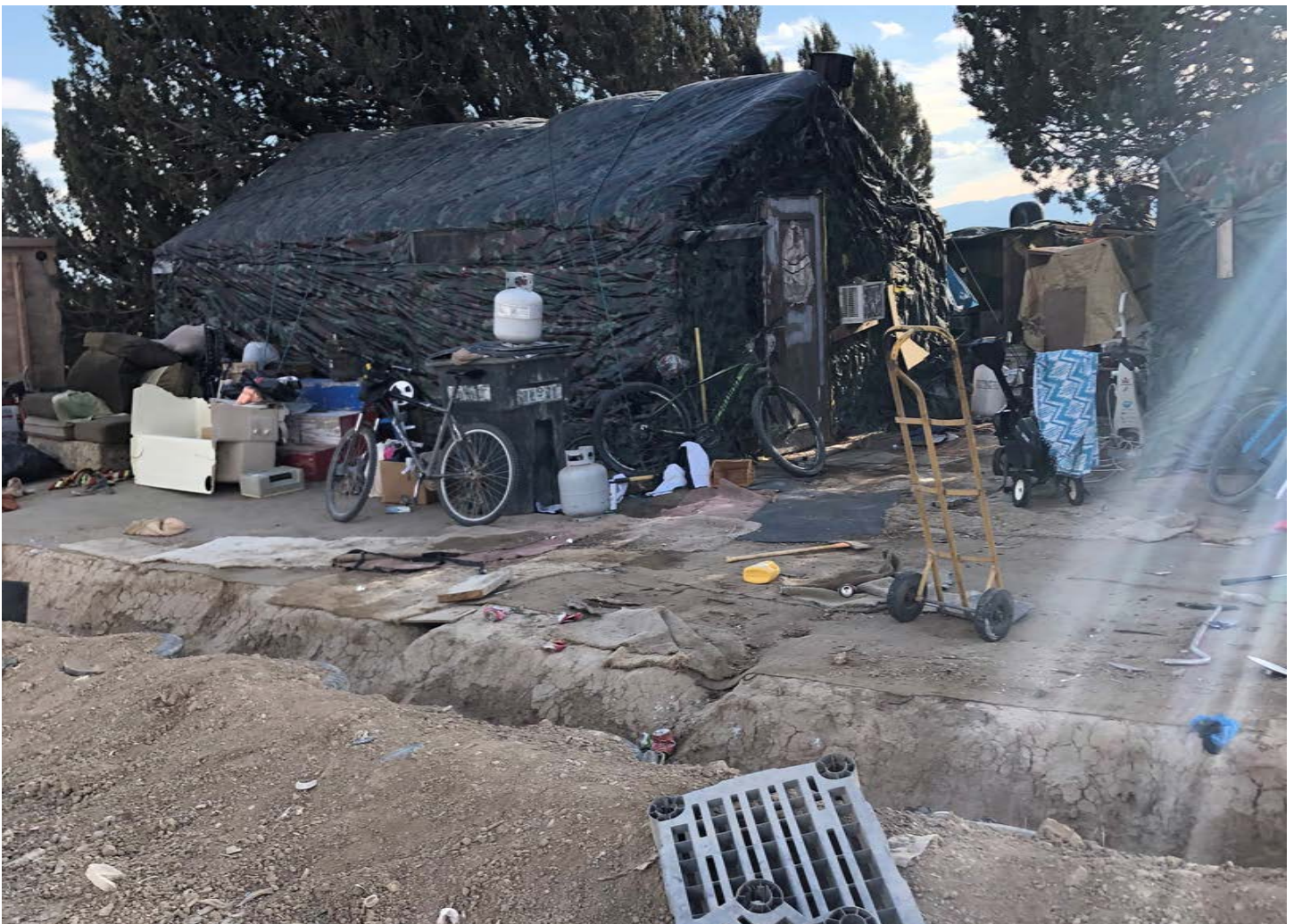
Structure built by residents of an encampment outside of Lancaster city limits.
